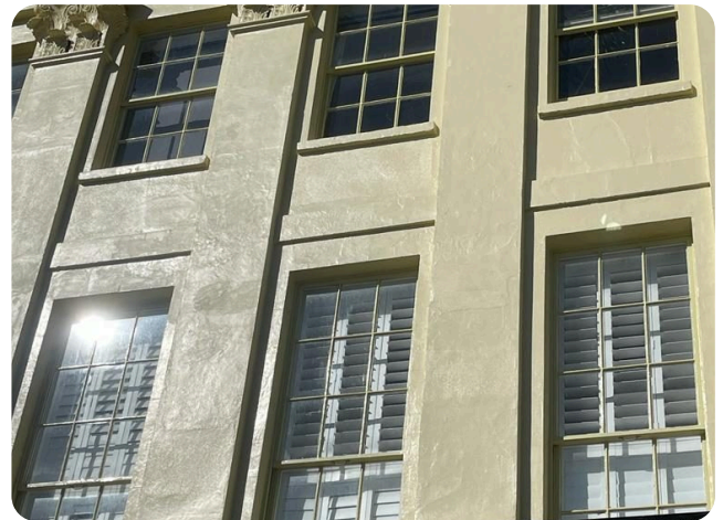
Facade detail: restored Corinthian capitals and columns
